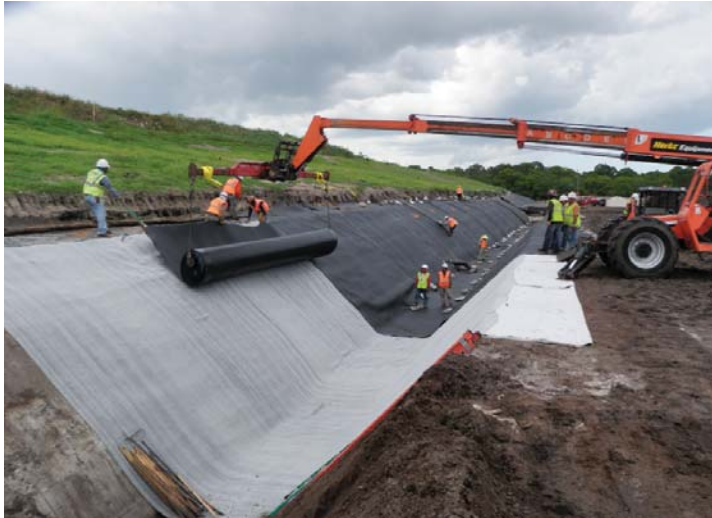
Geomembrane Liner Installation in LCT
