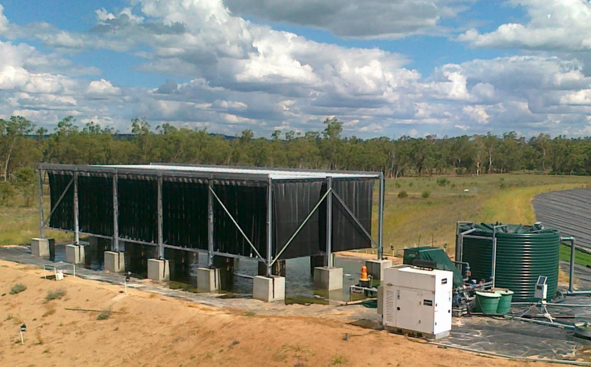
Supporting equipment (tank, pumps, filter, PLC, etc.)
