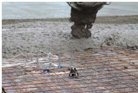
Instrumentation placed in concrete slab
