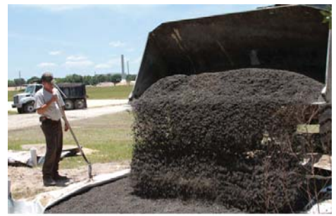
Ash base being placed in lined test patch
