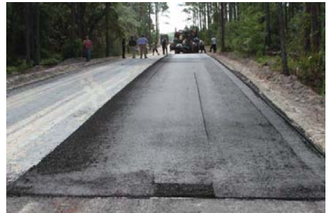
"Ash-fault" roadway construction
