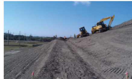
Photo 1 - Grading of tack-on berm and swale during construction.
