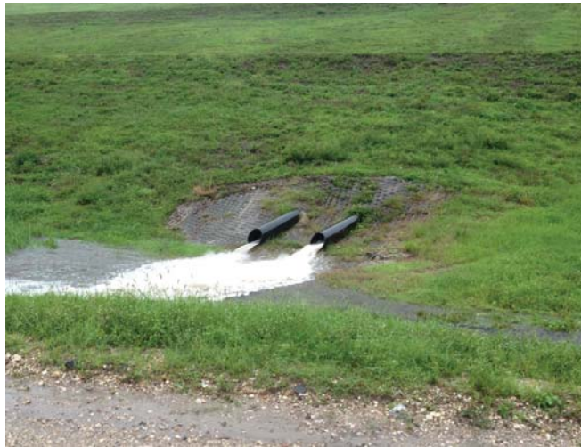
Photo 3 - Discharge points of downchute pipes.
