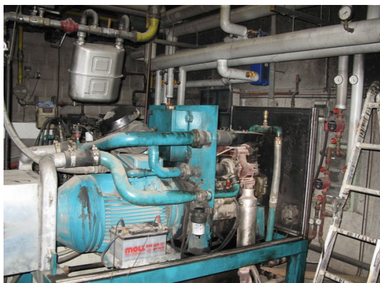
CHP (Combined heat and power) engine to generate electricity and heat from biogas.
