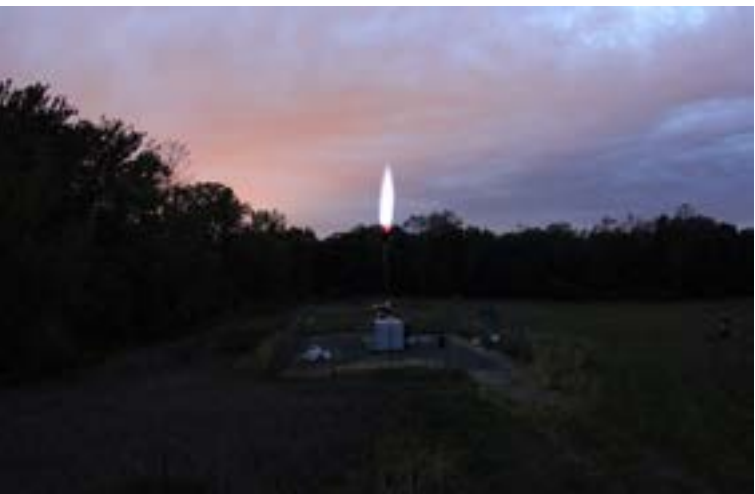
Simple LFG flare system. Photo courtesy of Vince Reinhart, CC BY-SA 2.0, via Wikimedia Commons.
