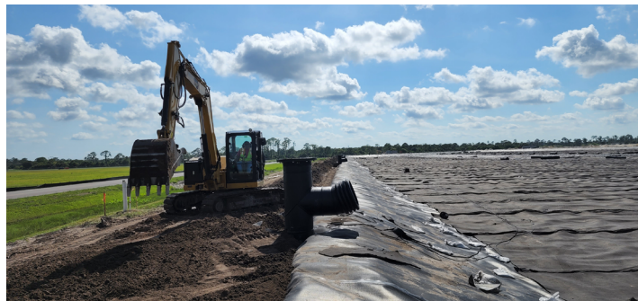
Permanent stormwater downcomer connection points.
