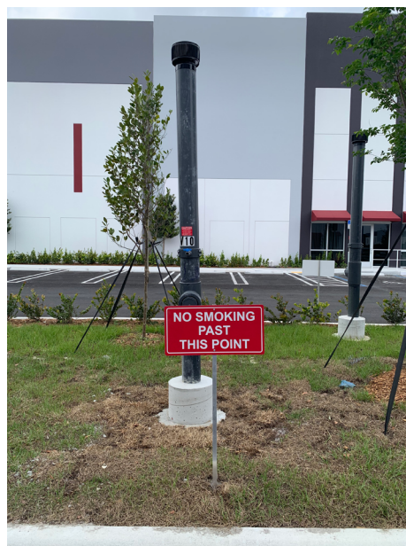
Passive Gas Vent Riser (typ.)
