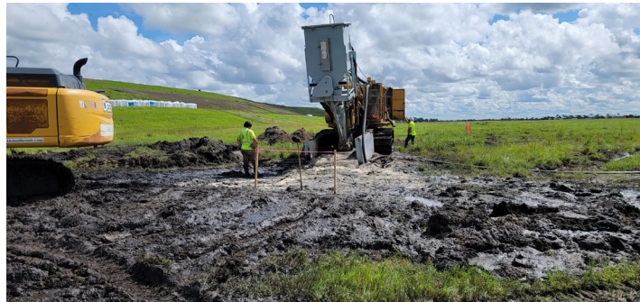
Installing slurry wall.
