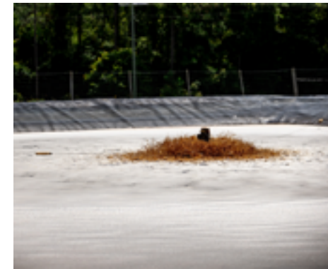
Untreated/Raw Leachate Aeration and Storage.
