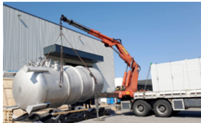
Delivery of the cryogenic distillation column.
