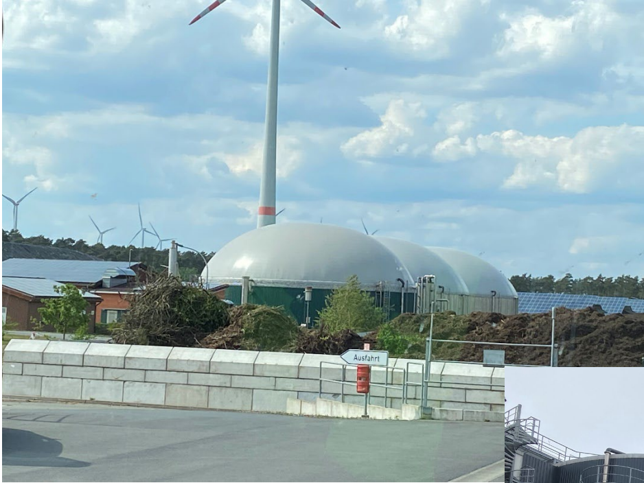
Saerbeck Bioenergy Park, Germany
