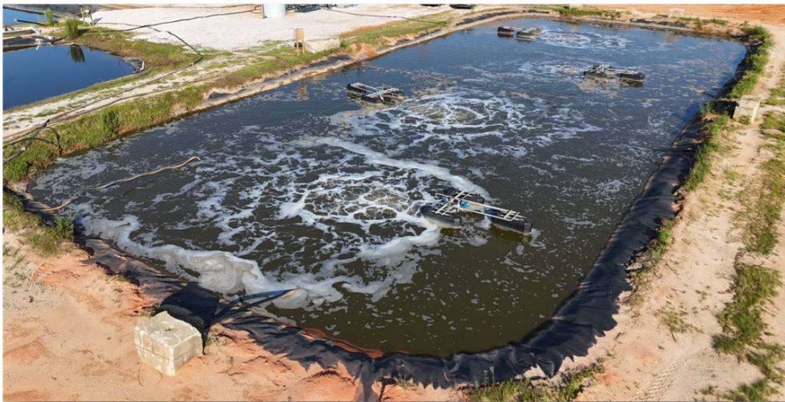
Bio-treatment Pond with Aerators Ammonia, BOD reduction
