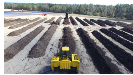
Equipment turning windrow piles.
